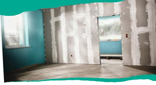
Now most of the hard work is done, you can focus on fine sanding. In order to achieve a smooth surface finish, the joints between the plaster boards in particular require thorough sanding with the hand-held grinder. Here it is important to make sure that the cardboard layer is not damaged. *wolfcraft* has developed the ergonomic 225 mm surface sander for quicker sanding progress and greater stability when working on walls.
