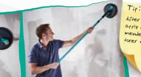
After sanding, you should apply a primer recommended by the manufacturer to the plasterboard.
