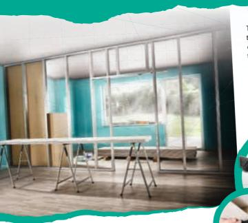
The stud frame has been erected, the plasterboard cut to the correct dimensions and the wall is slowly taking shape. You should provide a gap below the plasterboard adjacent to the floor. Universal wedges from wolfcraft are a worthwhile investment that will pay dividends in countless situations such as this.
