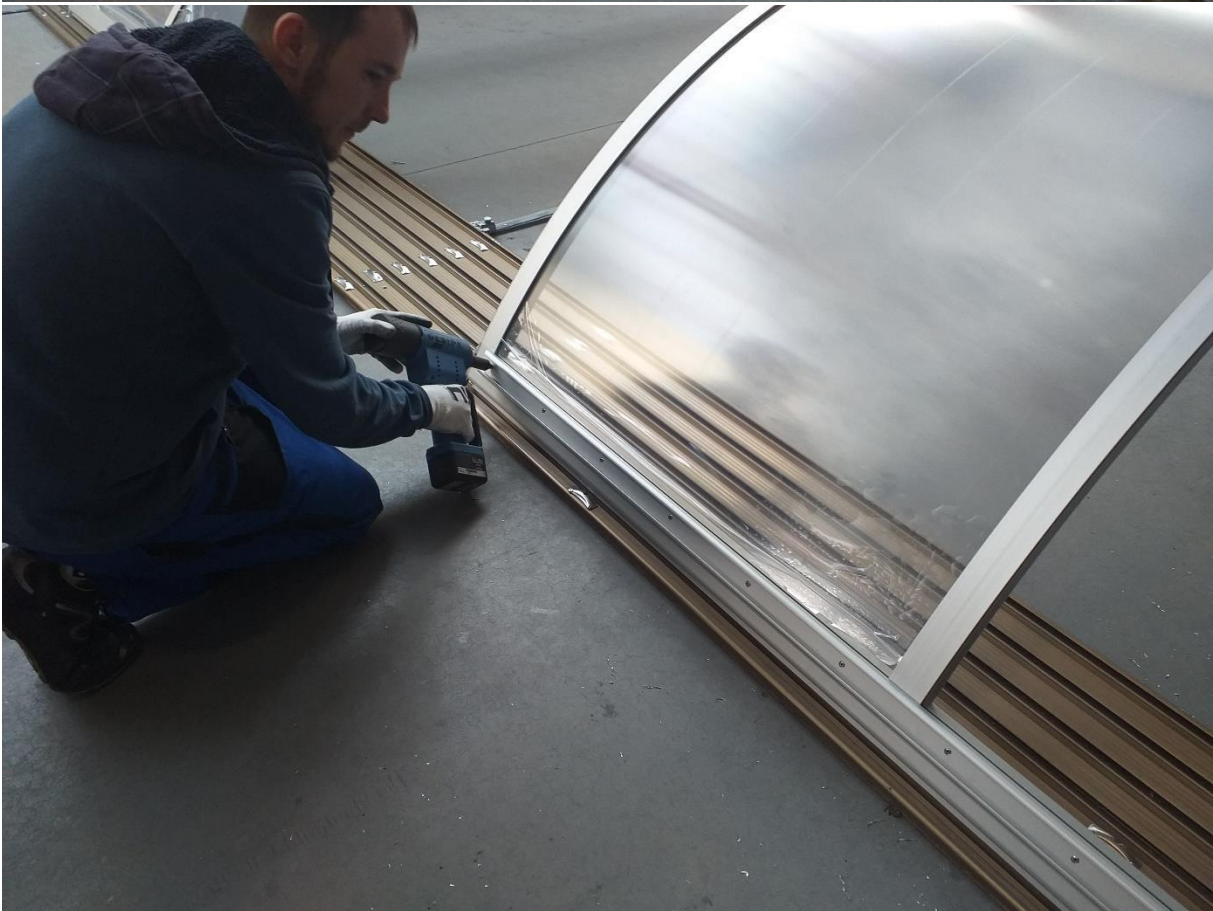
Final result after riveting:
